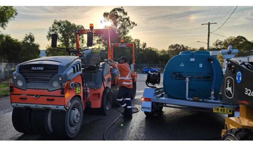
The WT2500 is a multi purpose, compact water cart trailer, designed to service multiple applications from dust suppression, slaking of binders, new subdivision hydration landscape care, fire fighting and equipment wash downs.
