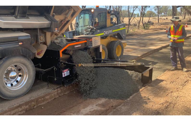
The ShoulderMaster SM2100 is a skidsteer/wheeled loader shoulder paving attachment that can increase the road shoulders from 19"out to 7ft 5" wide.
